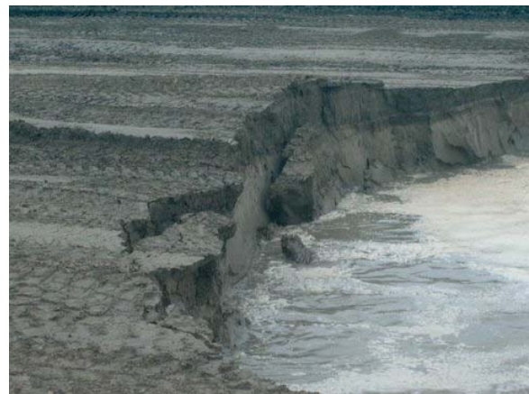
Sand Breaking Off as Dredge Advances
