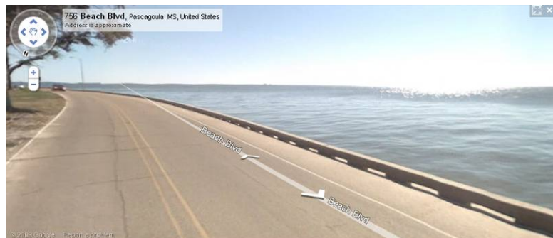
Google Satellite Image- Before the beach was created, the existing sea wall provided the only protection to Beach Boulevard.
