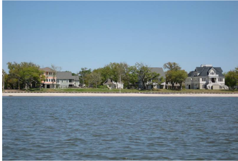
The newly created beach is 1.5 miles long and ties into an existing beach, providing added storm protection to the seawall and aesthetics to the area.
