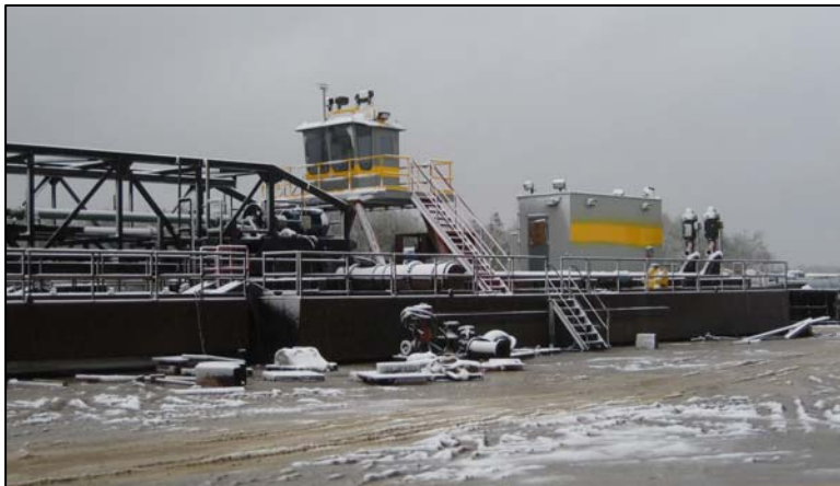
A rare dusting of snow in Reserve, Louisiana covers the lever room, electrical room and equipment.
